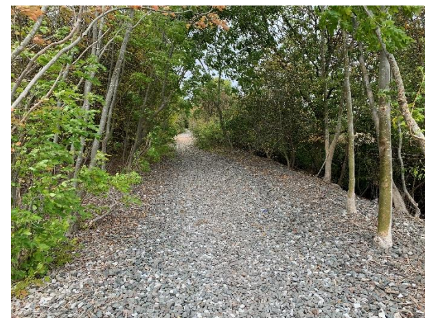
Fig 20 Clearer and heavily ballasted railway corridor at the southern end.
