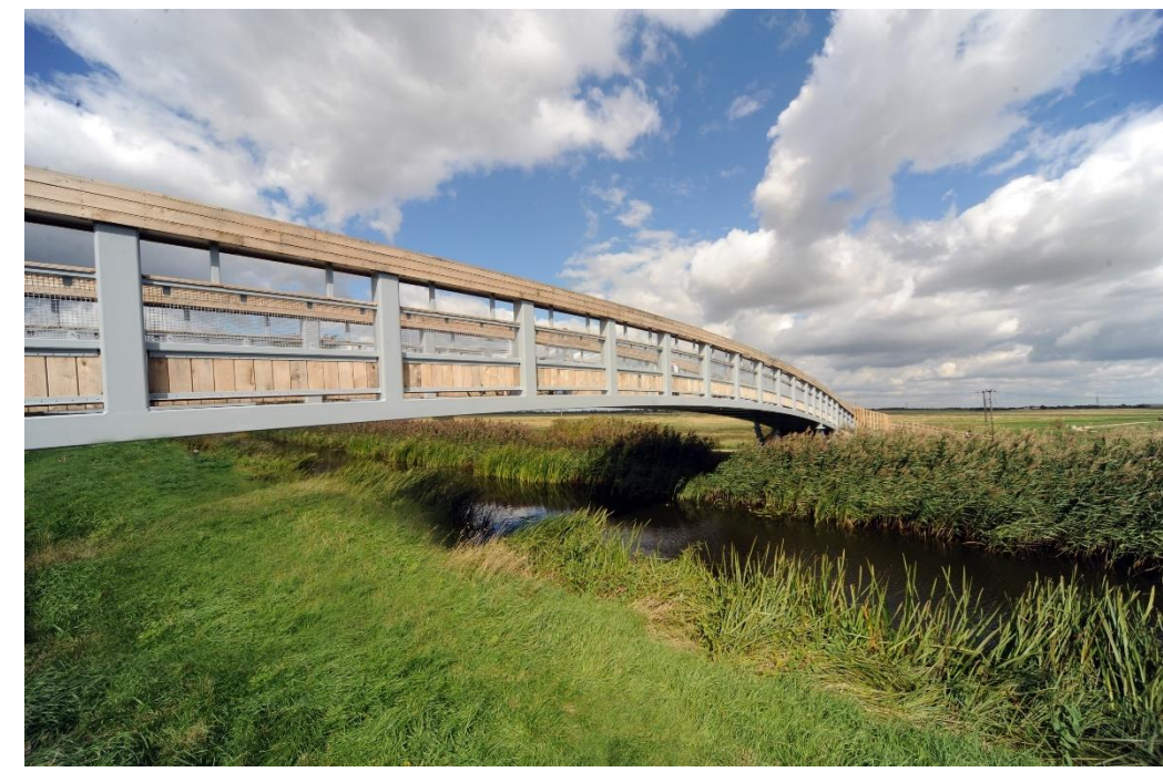
Fig 55 Any new structure needs to blend into the landscape – this is Reach Lode bridge in Cambridgeshire
