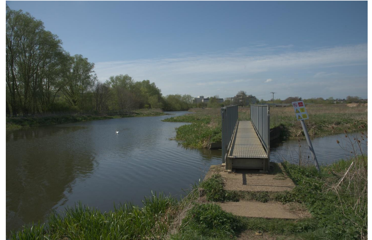
Fig 01 Existing bridge over the creek on the River Nene, inaccessible for many potential users.
