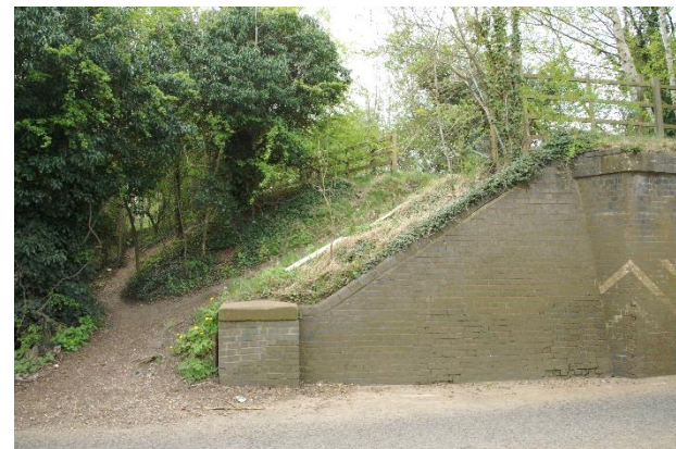
Fig 19 Railway bridge abutments and clearly formed access tracks onto the old railway.
