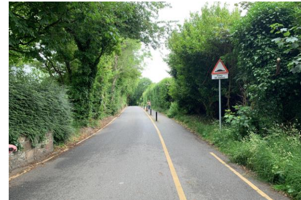
Bollards spaced intermittently along quieter rural roads can provide protected space for vulnerable users (Jersey)
