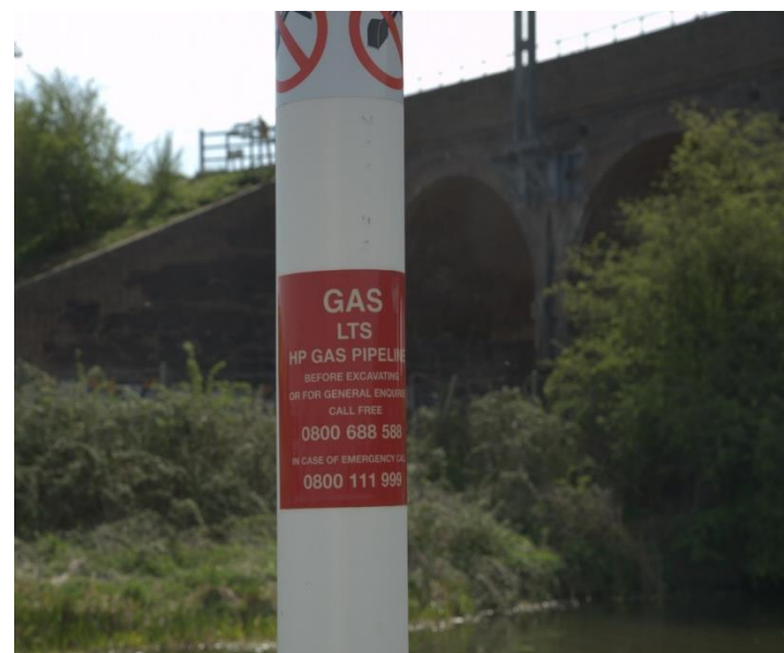
Fig 50 Local High-Pressure gas main needs to be considered in any design and construction conversation.
