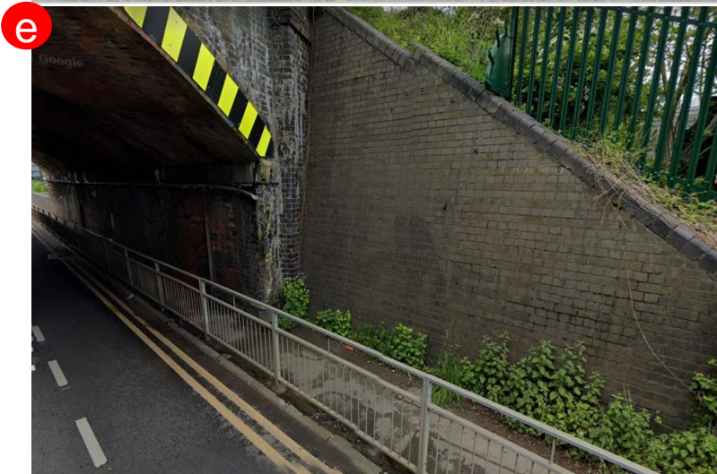
Narrow footpath under bridge.
