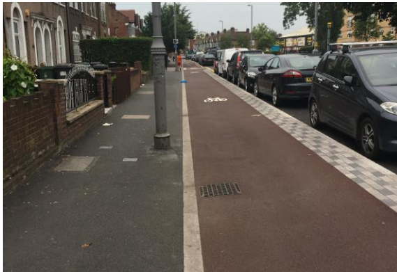
Constructing cycle tracks at (or close to) footway level can be a good solution where space is very constrained (Waltham Forest)
