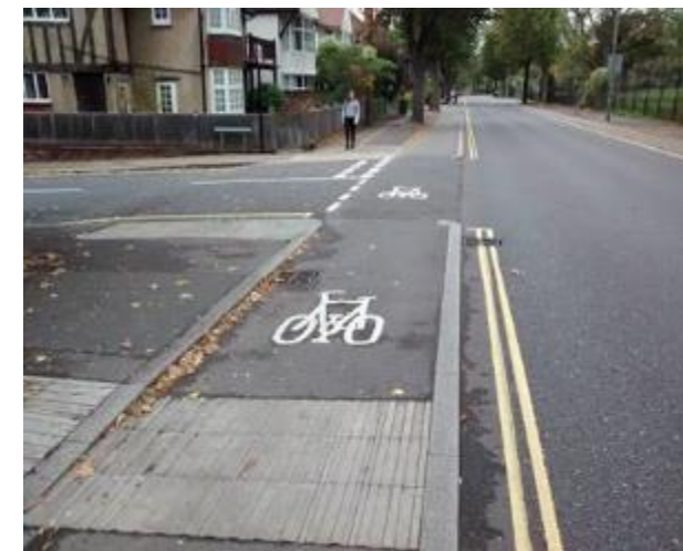
Figure 5: At grade crossing of side road with separation for traffic, cyclists and pedestrians
