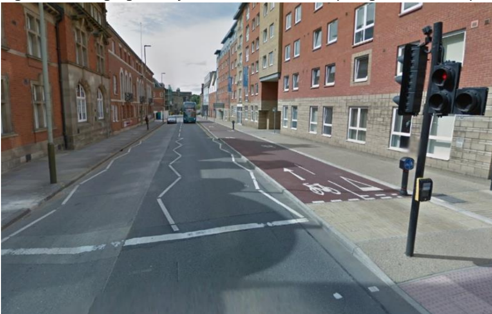
Figure 4-7 – Segregated Cycle Track in Leicester (Google Street View)
