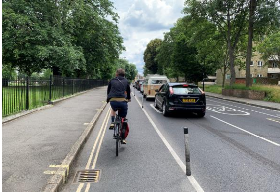
Light segregation using flexible bollards is a cost-effective way of created protected space for cycling (Green Lanes)
