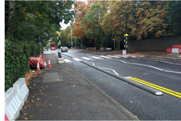
Bolt-down kerbs which can look less visually intrusive than wands are another option for creating cycle tracks (Kingston Hill)
