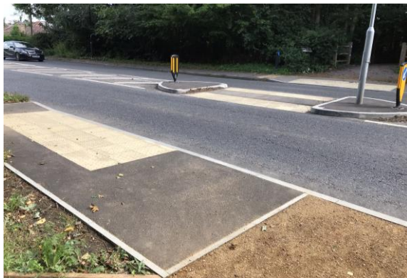
Uncontrolled crossings with wide central refuges can be used where signal controlled crossings are not appropriate (Burgess Hill)
