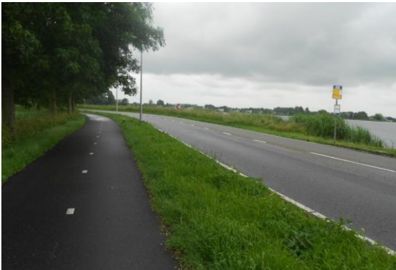
A dashed centre line on a shared footway/cycleway can help remind users to keep to the left to minimise conflict (Netherlands)
