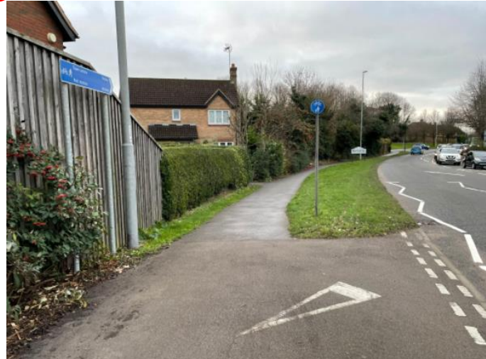
Contradicting signage and markings on Rockingham Rd (S1)
