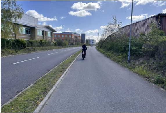
Shared use footways/cycleways should have a buffer to the carriageway where possible, especially on faster roads (Cambridge)
