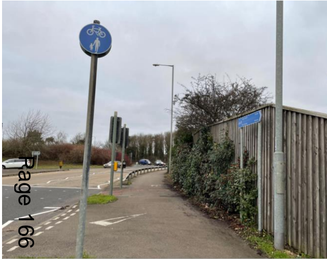
Rockingham Road looking north at the A43 / A6183 roundabout (J1)
